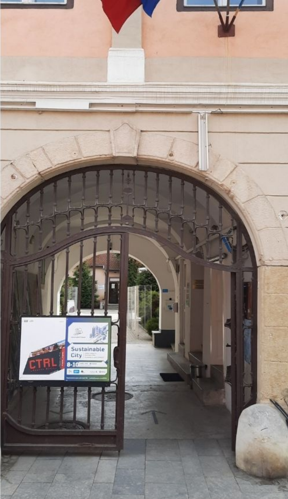
Entrance Bratianu building
