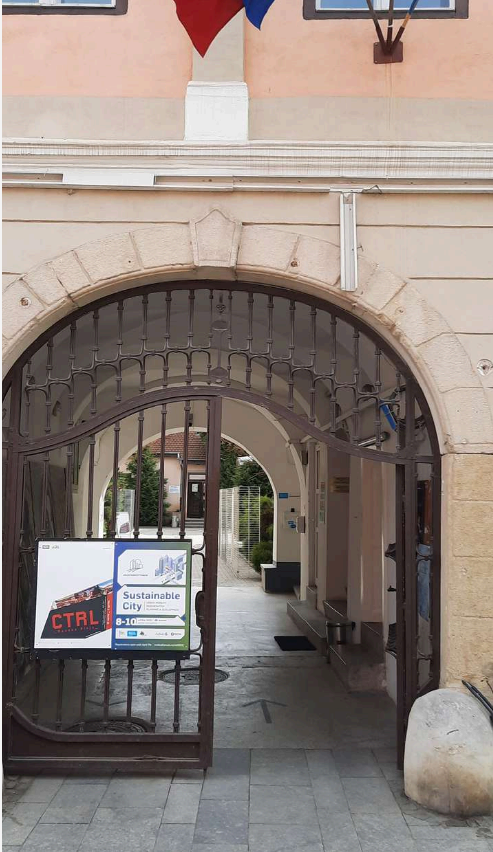
Entrance Bratianu building
