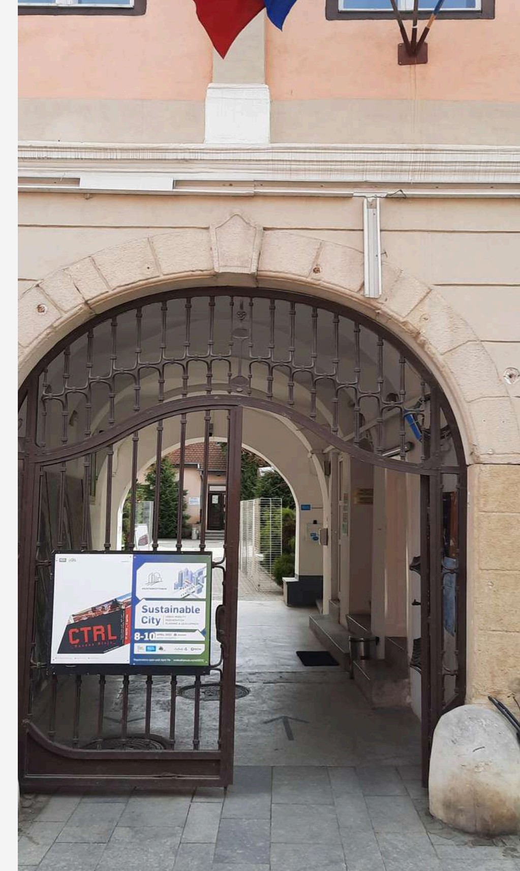
Entrance Bratianu building
